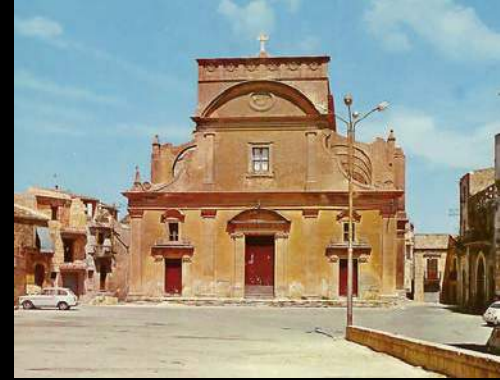
Cathedral of Salemi, before the earthquake
